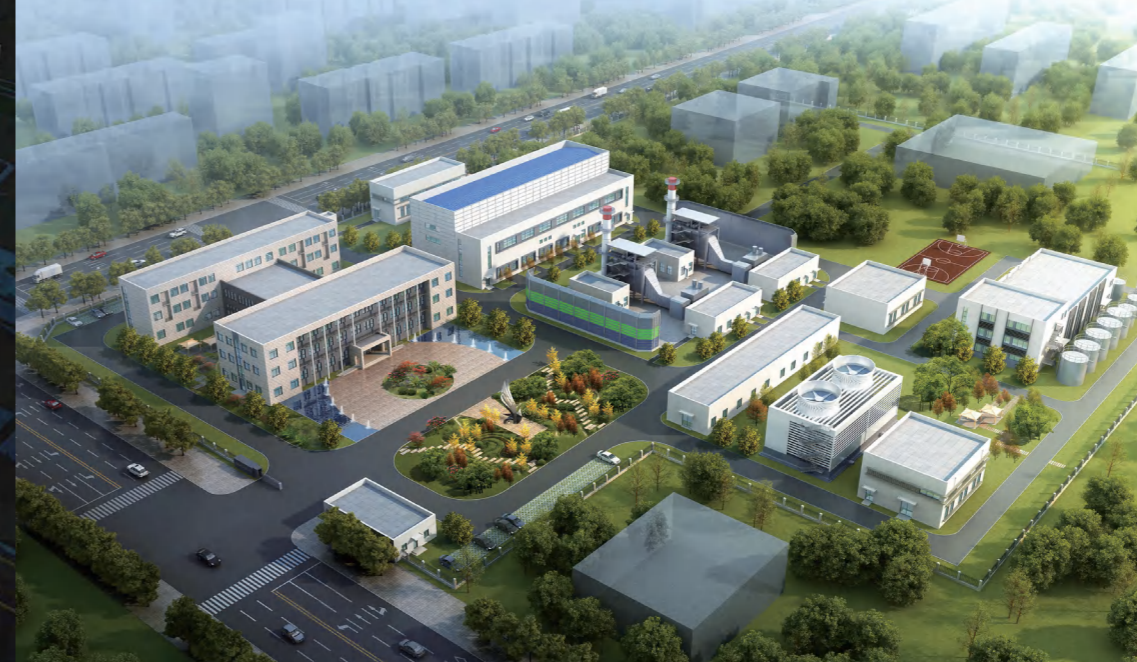
▲ Gas-Steam Combined Cycle Cogeneration Project of Shandong Qingdao Gaoxin Thermal Power Co., Ltd.
