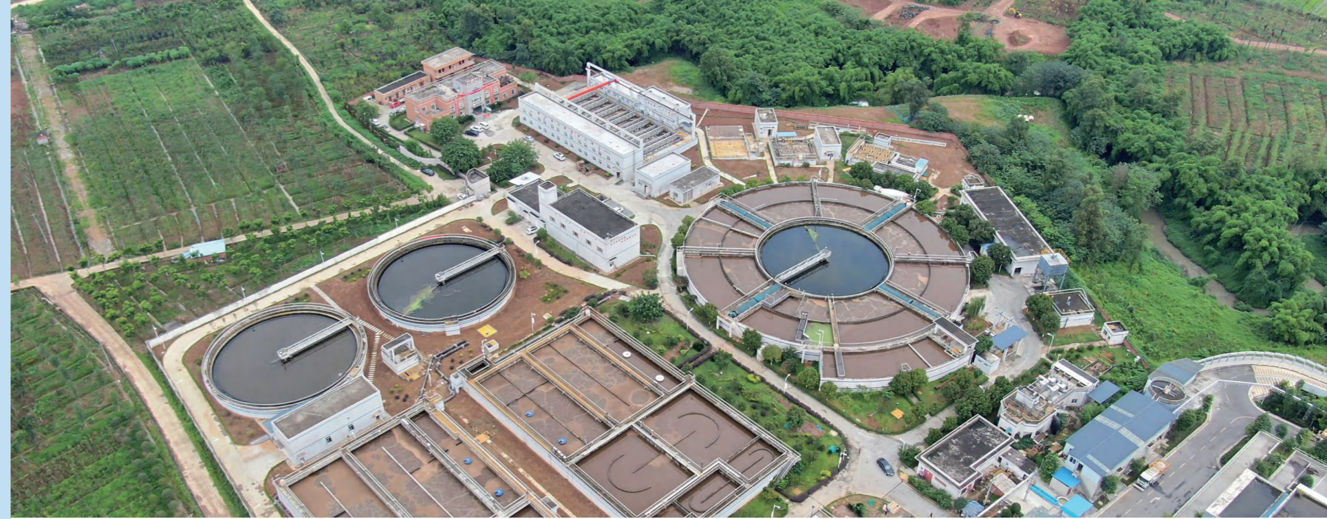
▲ Sewage Treatment Plant, BOT project in Longquanyi District, Chengdu, Sichuan Province ▼ Anren Sewage Treatment Plant, BOT project in Dayi County, Chengdu, Sichuan Province
