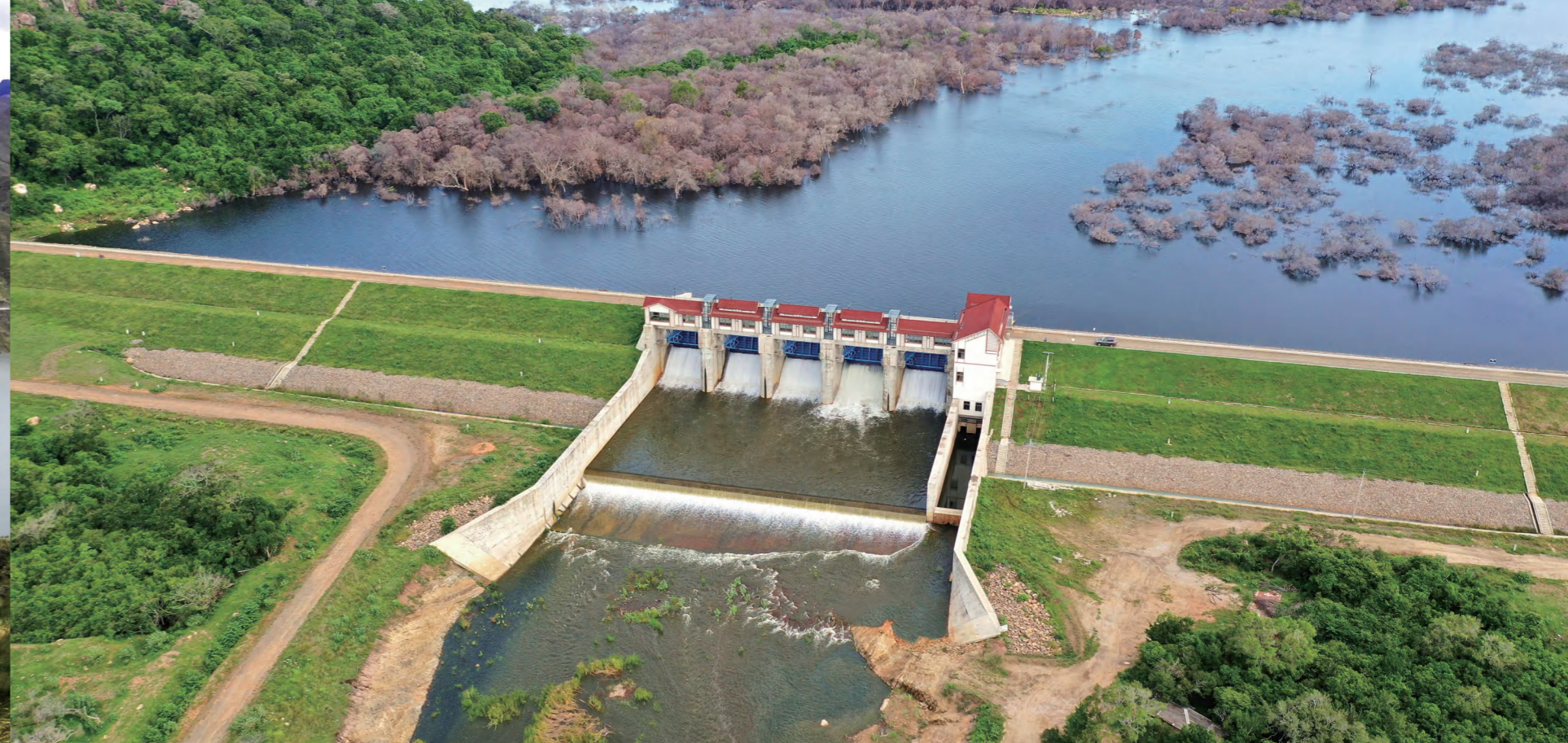
▲ Yan Oya Reservoir Project in Sri Lanka (Dam height 20m, Reservoir capacity 200 MCM)
