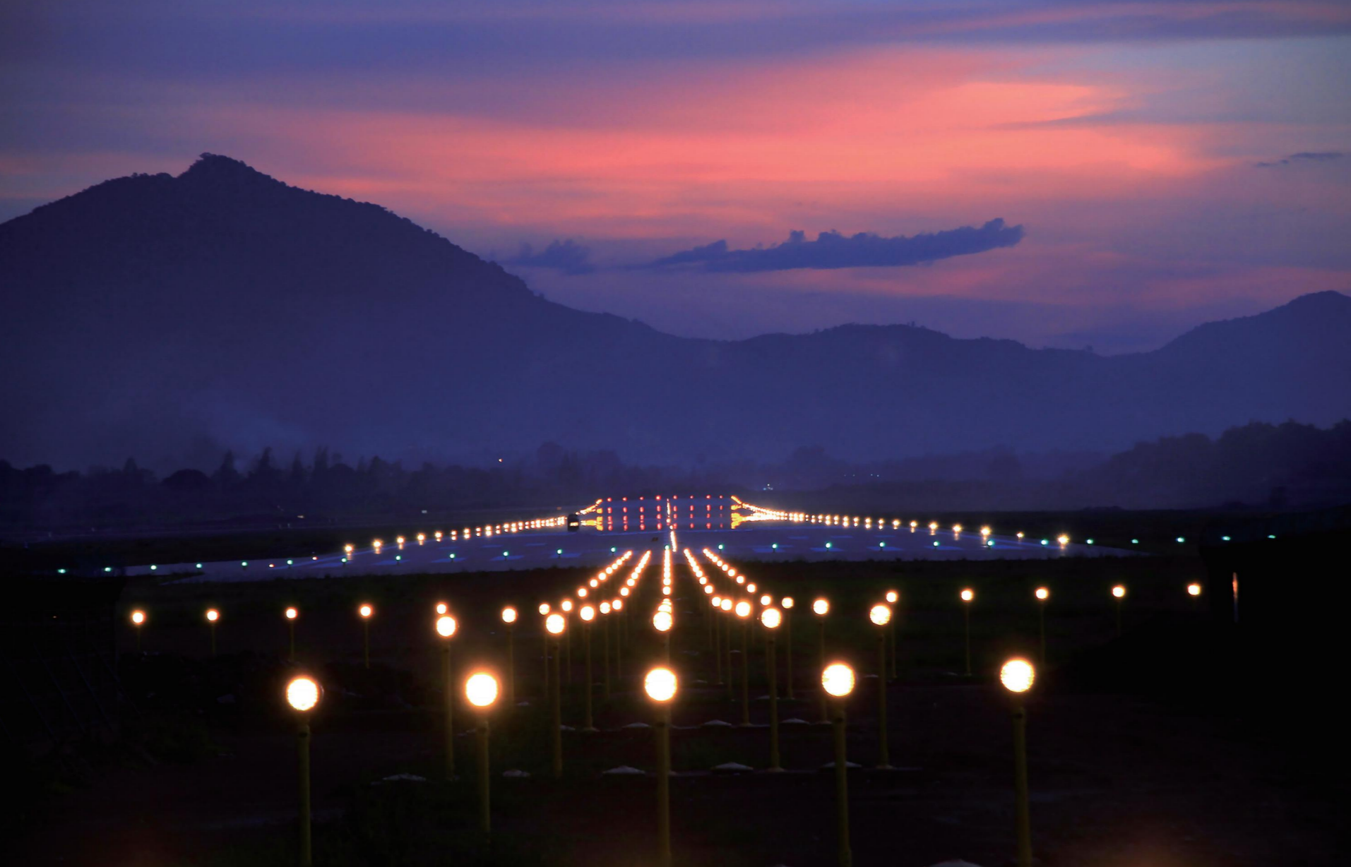
▲ Reconstruction of Luang Prabang International Airport in Laos ( This project includes the terminal, runway, flight procedure devising etc.)
