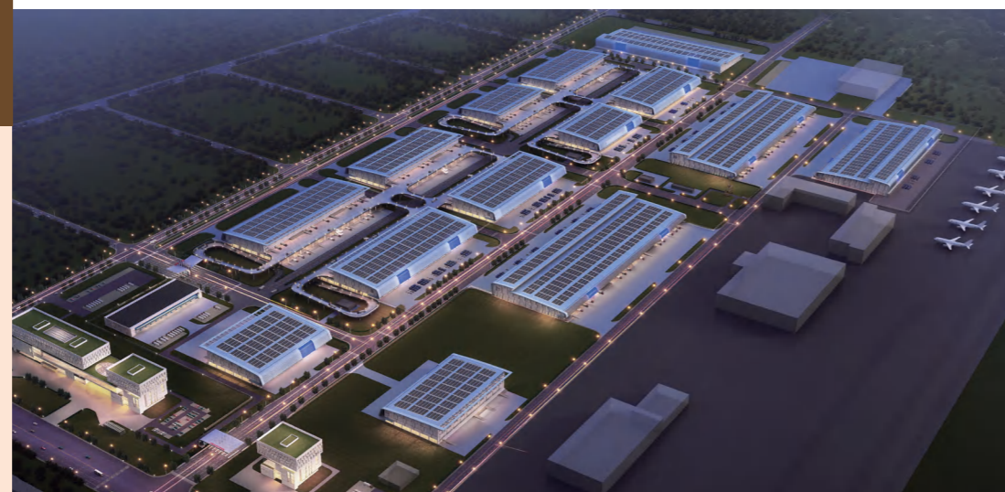
▲ Project of the Clearance Depot of Tianjin Airport (Phase I)
