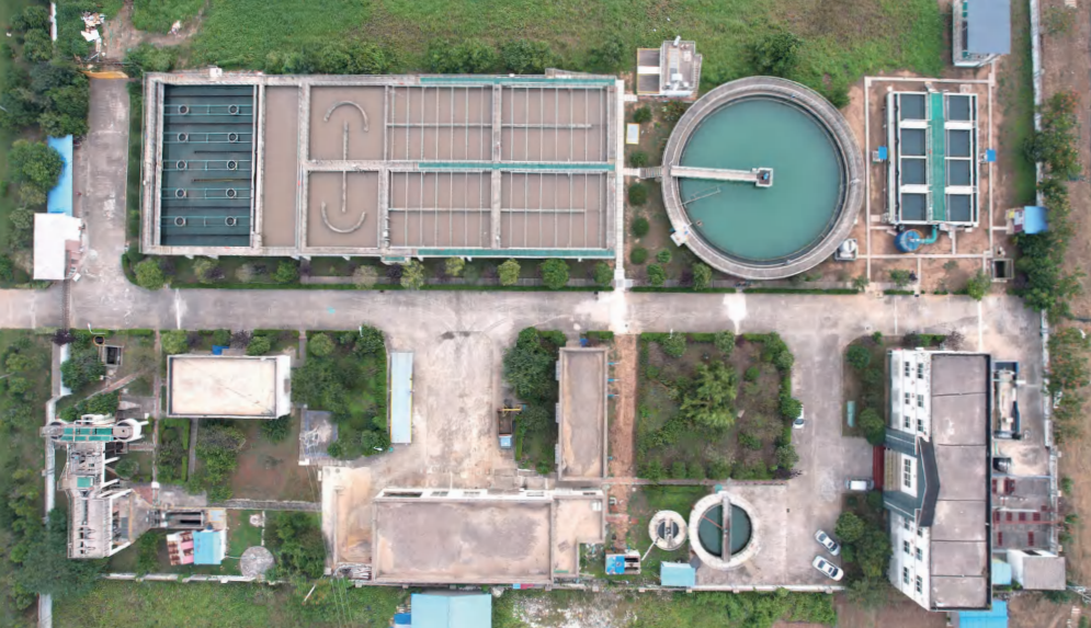
▲ East City (Paoche) Sewage Treatment Plant, TOT project in Pizhou, Jiangsu Province
