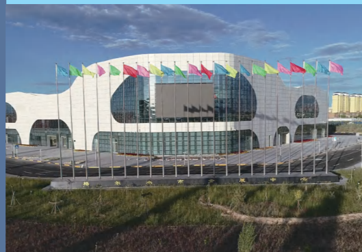
▲ Golmud Exhibition Center project
