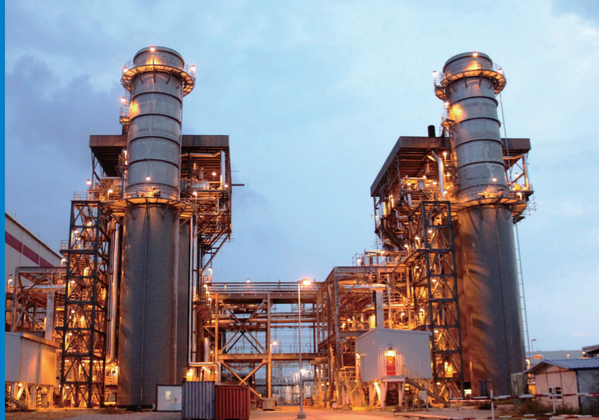
▲ Don Luis Zambrano Combined Cycle Power Plant in Venezuela (Total installed capacity 597MW based on the ISO case consuming natural gas )
